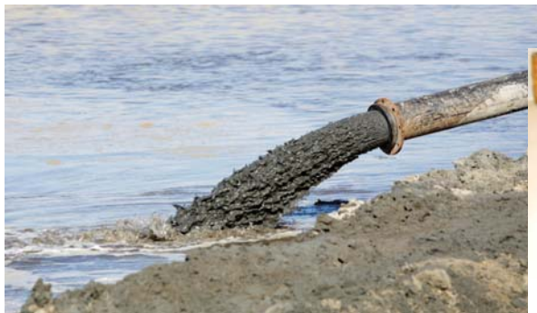
Sediment "slurry" from hydraulic dredging.
